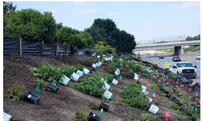
Once established, diverse plantings along sloped freeway roadsides can reduce runoff and erosion with little maintenance.
