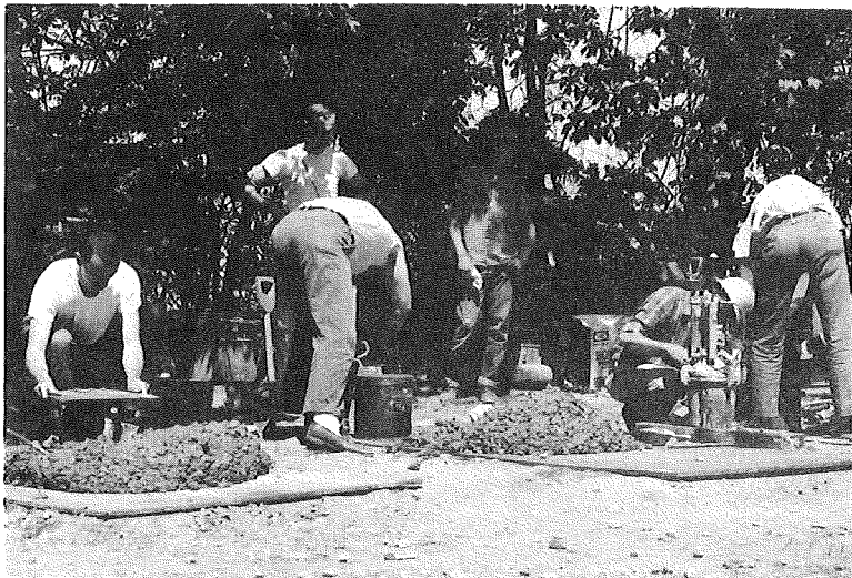
Unit weight and pressure air testing
