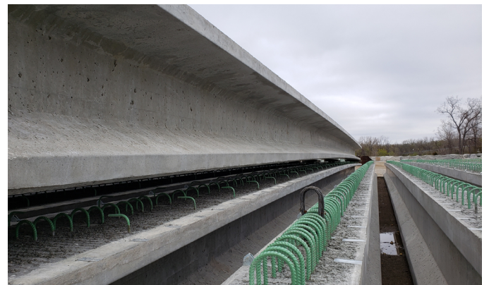
Prestressed concrete beams stored in a fabricator's yard display a slightly arched shape, or camber.
