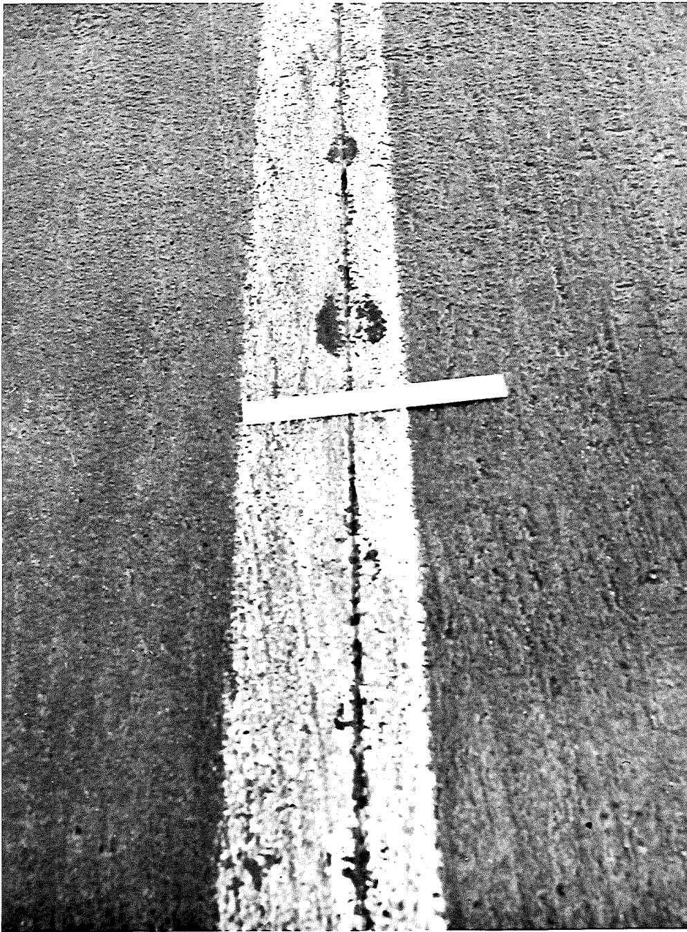
▲ FIGURE 1. SAWED LONGITUDINAL JOINT AT WHITE PAINT STRIPE ▲ FIGURE 2. SAWED LONGITUDINAL JOINT AT BLACK PAINT STRIPE US-31 HOLLAND BY-PASS. STATION 212 + 50 S.B.
