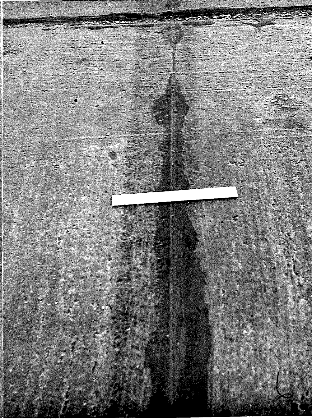
▲ FIGURE 1. SAWED LONGITUDINAL JOINT AT WHITE PAINT STRIPE ▲ FIGURE 2. SAWED LONGITUDINAL JOINT AT BLACK PAINT STRIPE US-31 HOLLAND BY-PASS. STATION 212 + 50 S.B.
