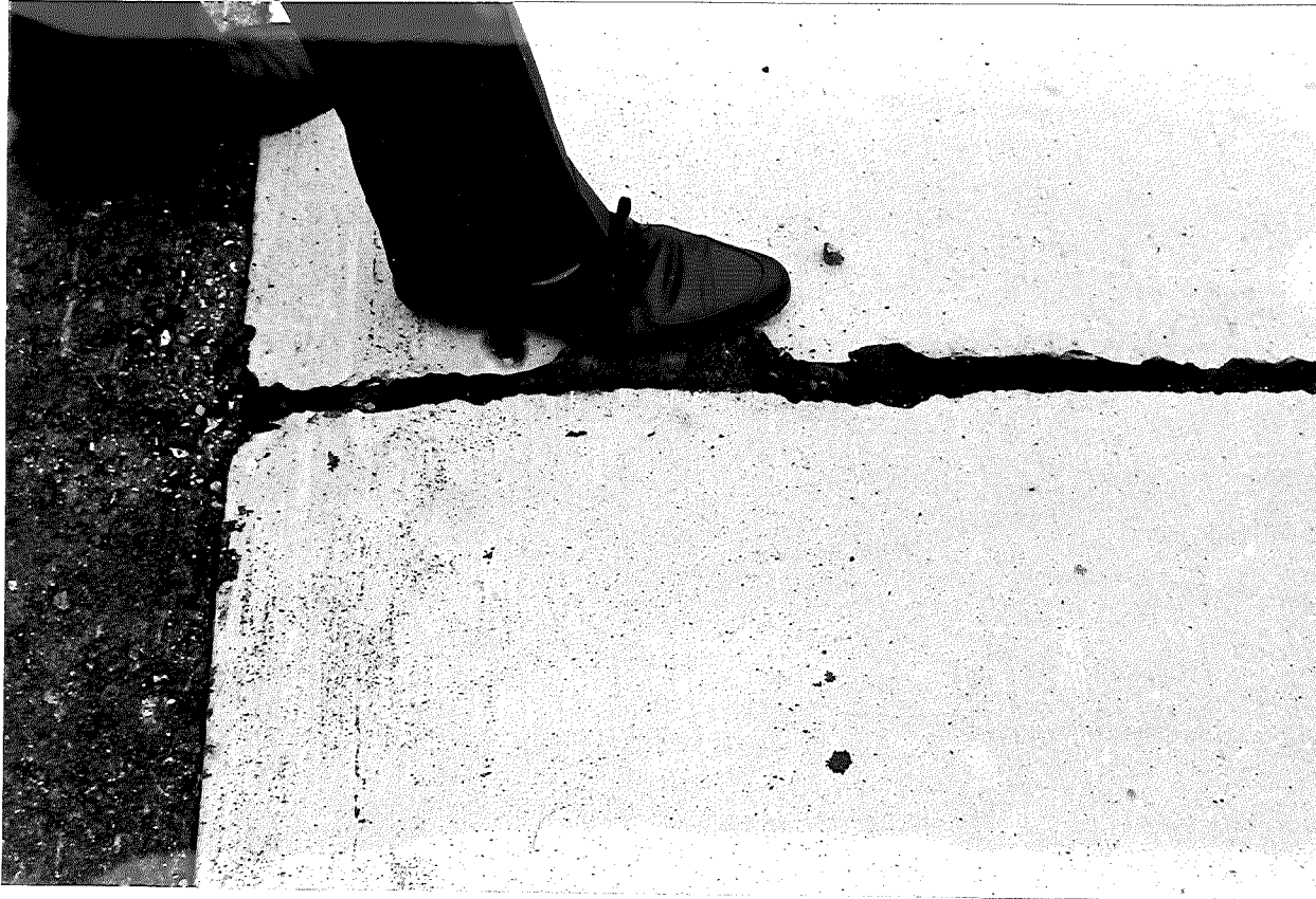
Figure 2. Adhesion failure with dirt infiltration, preventing good bond of sealant to joint face when joint narrows in warm weather (Sta. 537+30 SB, June 1964).
