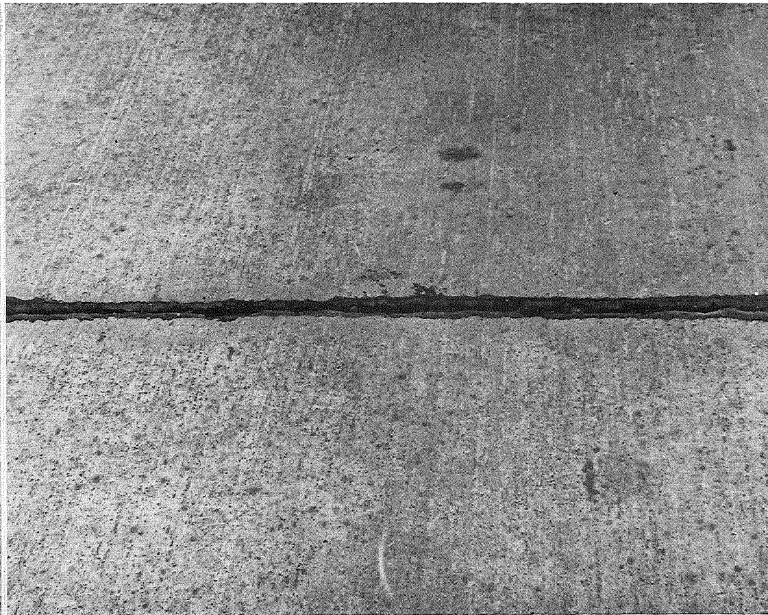
Figure 1 (left). Typical adhesion failure with sand and gravel embedded in joint seal (Project BI 50111 I, C12, Sta. 87+70 SB).
