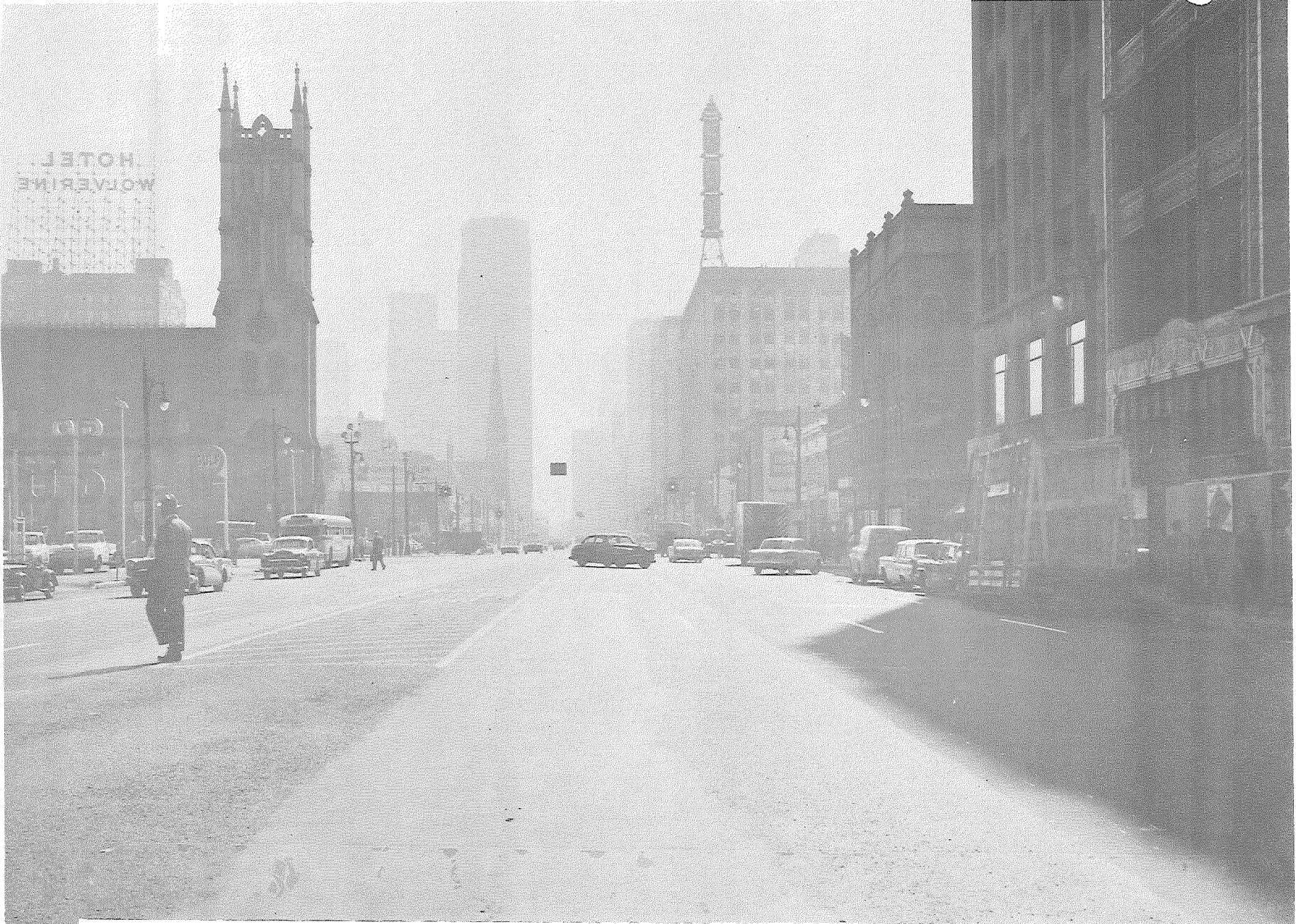
Figure 2 - View of Signals at Intersection of Woodward and Montcalm Looking South from Winder Intersection
