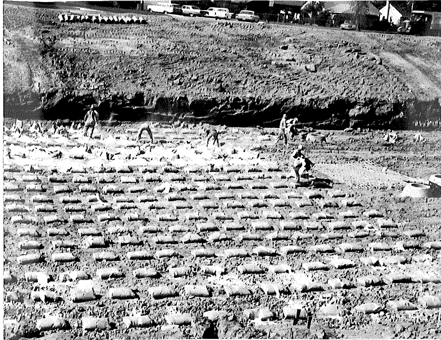
Figure 1. Spotting and spreading of bagged lime.
