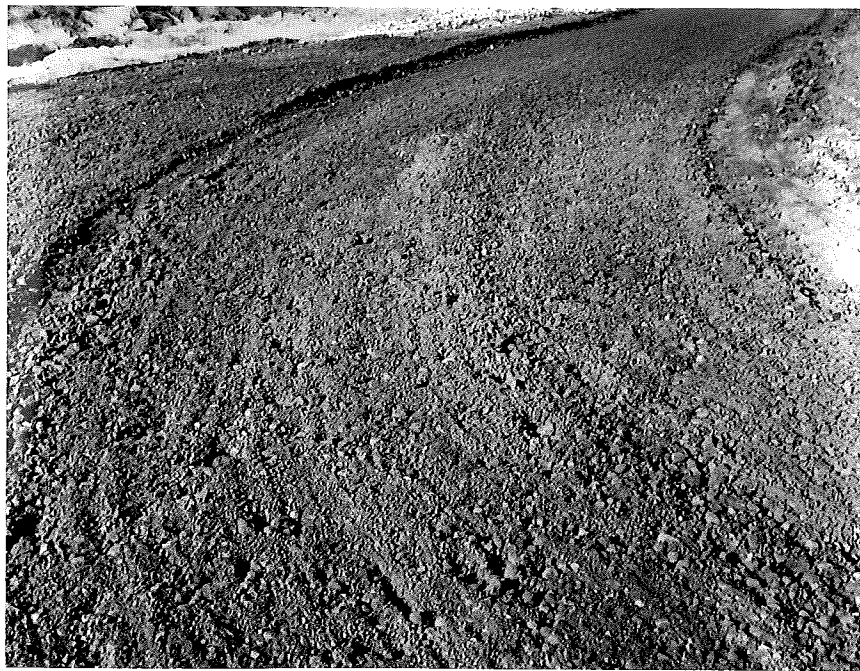
Figure 6. Close-up of mixture prior to compaction.
