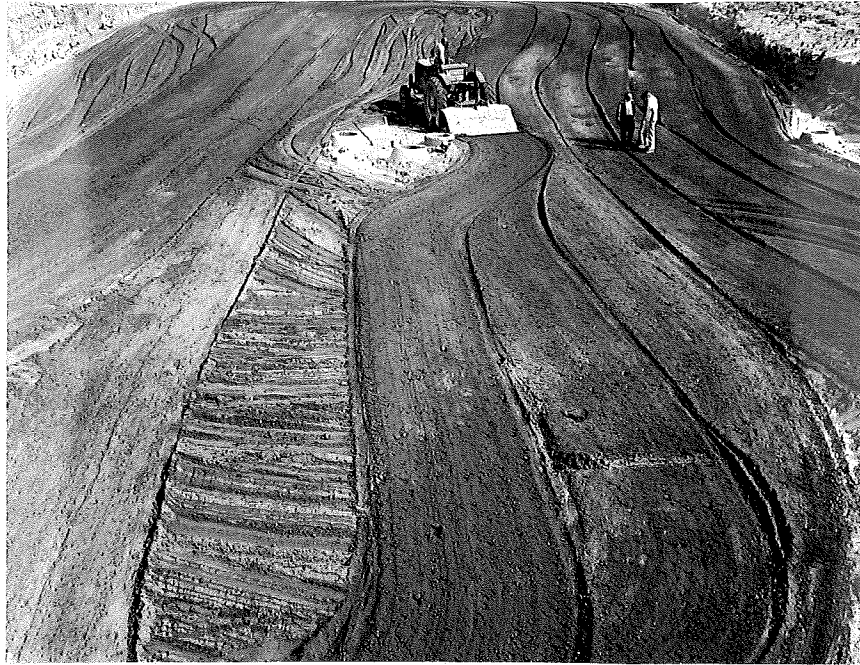
Figure 5. General view prior to compaction.
