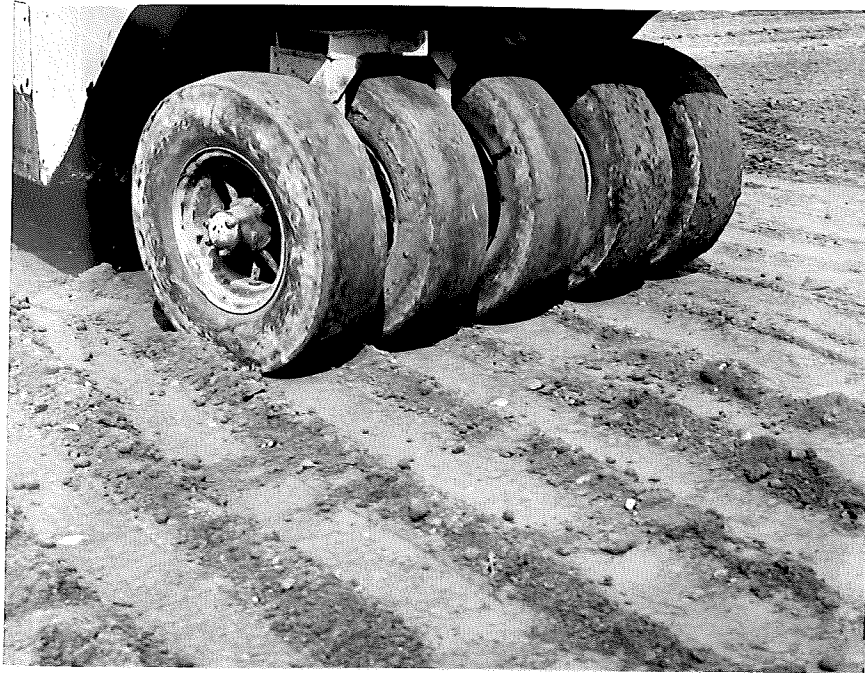
Figure 7. Compaction with rubber-tired roller.
