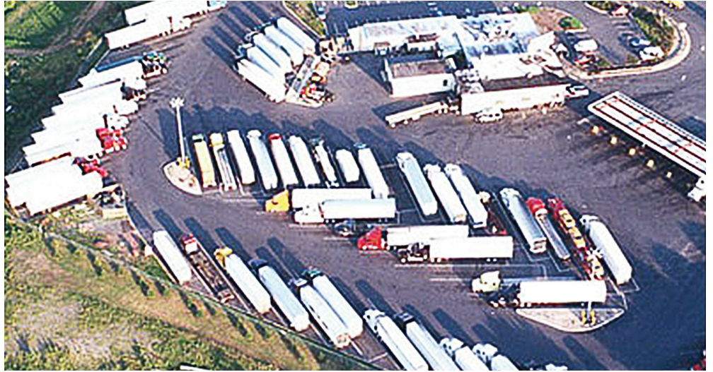
MDOT is piloting a truck parking information and management system (TPIMS) on I-94. The system will alert drivers to available truck parking spots through a variety of electronic systems and signs.
