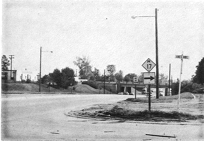
Figure 4. Looking south on US 24 at the intersection with M 17 N Jct (Ames Hwy) (left), signs and utility poles interfere with visibility. At the US 24 centerline directly north of the Ames Highway intersection (right), the truck turning from M 17 at right blocked southbound traffic.
