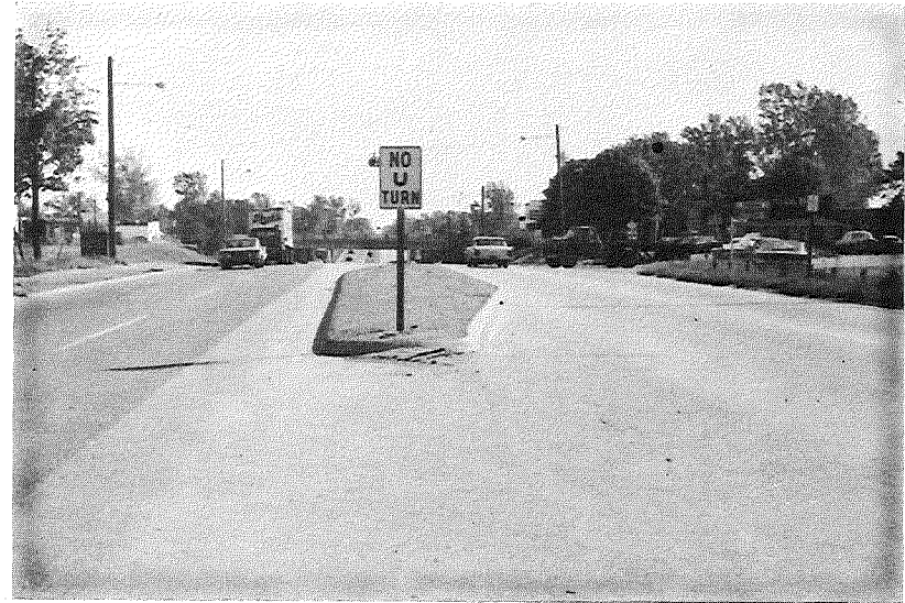
Figure 4. Looking south on US 24 at the intersection with M 17 N Jct (Ames Hwy) (left), signs and utility poles interfere with visibility. At the US 24 centerline directly north of the Ames Highway intersection (right), the truck turning from M 17 at right blocked southbound traffic.
