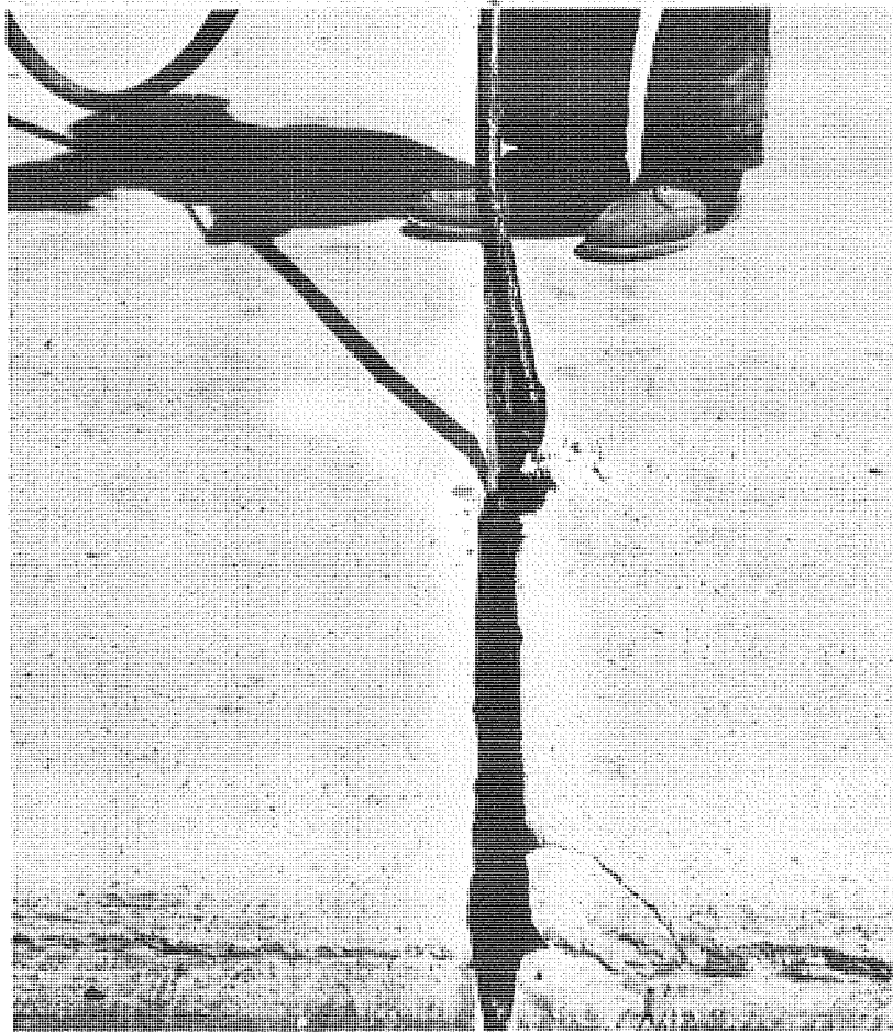
Figure 6. Barton used truck-mounted melter-applicator.
