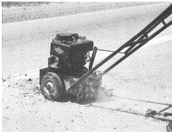
Figure 4. Young also used Windsor router (left) and then scarified with an abrasive saw (right).
