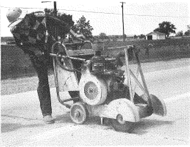
Figure 4. Young also used Windsor router (left) and then scarified with an abrasive saw (right).
