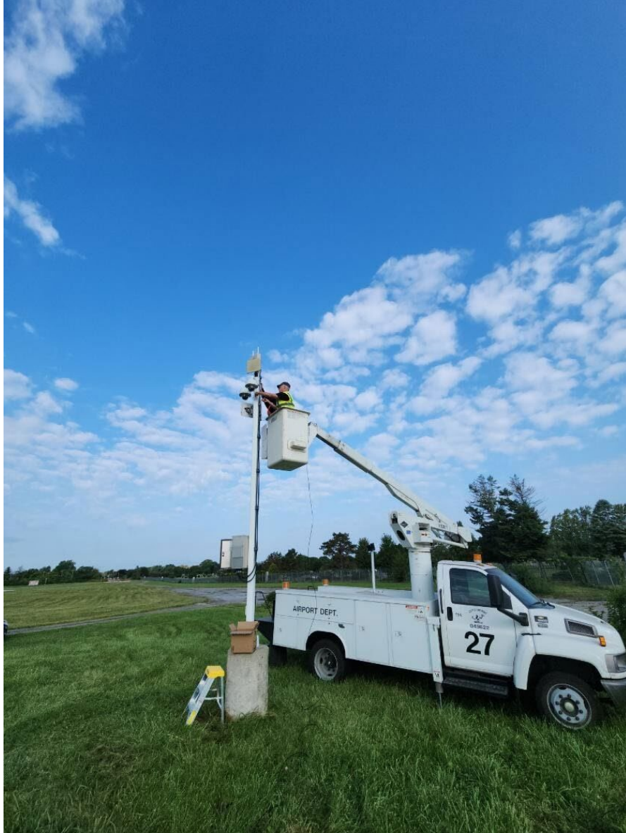
FIGURE 18. EQUIPMENT INSTALLATION AT DET
