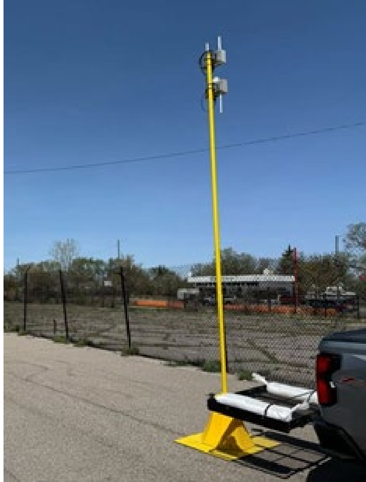
FIGURE 28. TEMPORARY RSU STAND WITH TWO RSUS - C-V2X TOP AND DSRC BOTTOM
