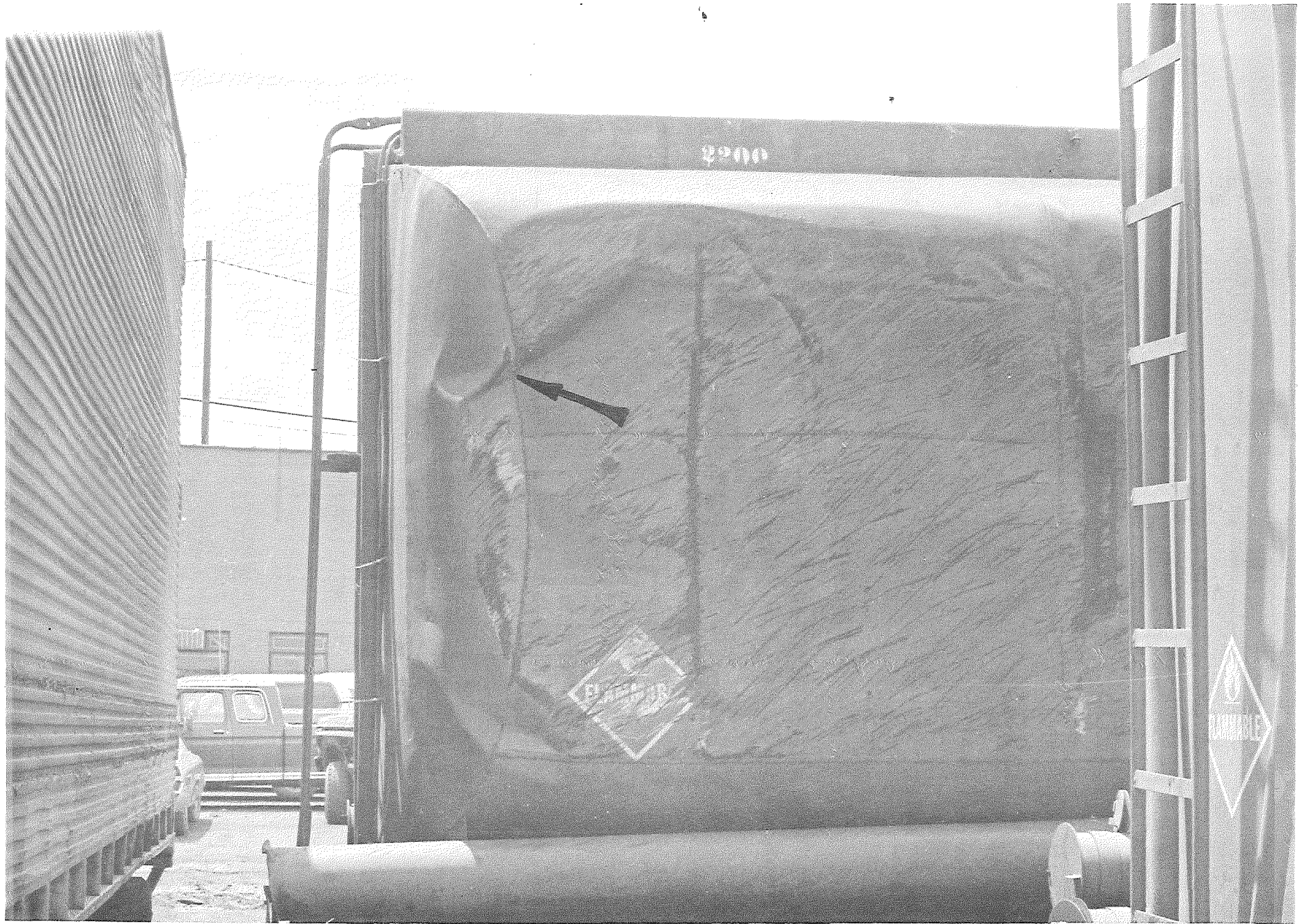
Figure 5.6. Side view of flattened tank wall with characteristic concave fold (arrow) such as commonly produces weld seam split.
