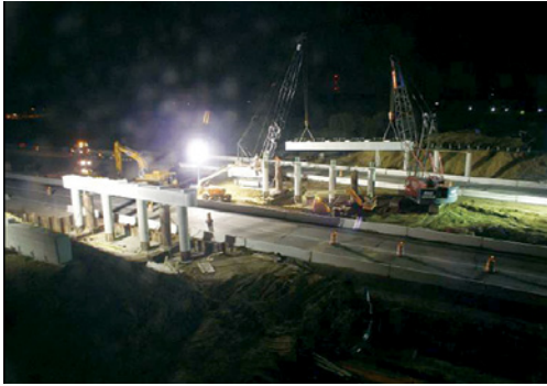
One of MDOT's three accelerated bridge construction projects to date involved replacing a bridge in 2009 on Parkview Avenue over US-131.
