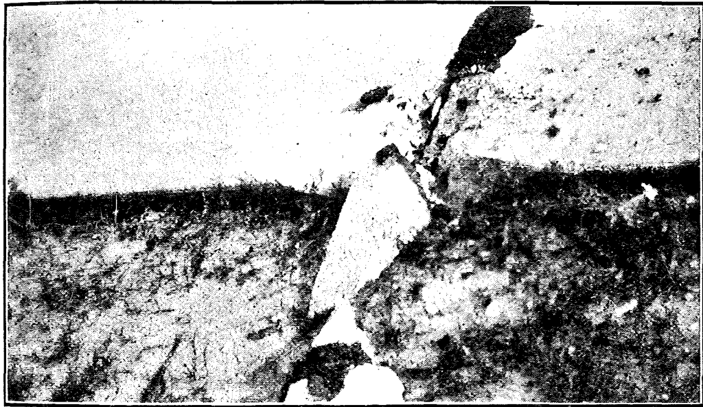
FIG. 2.—TYPICAL BREAK IN ROAD AT POINT OF ARC.
