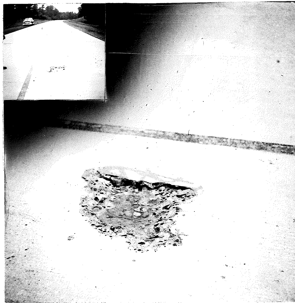
▲ FIGURE 7—U. S. 41. PICTURE TAKEN BY STATE POLICE EARLY ON MORNING, JULY 7 1951. NOTE RAGGED CONDITION OF SPALLED SURFACE AND WIRE REINFORCEMENT AT BOTTOM OF SPALL.
