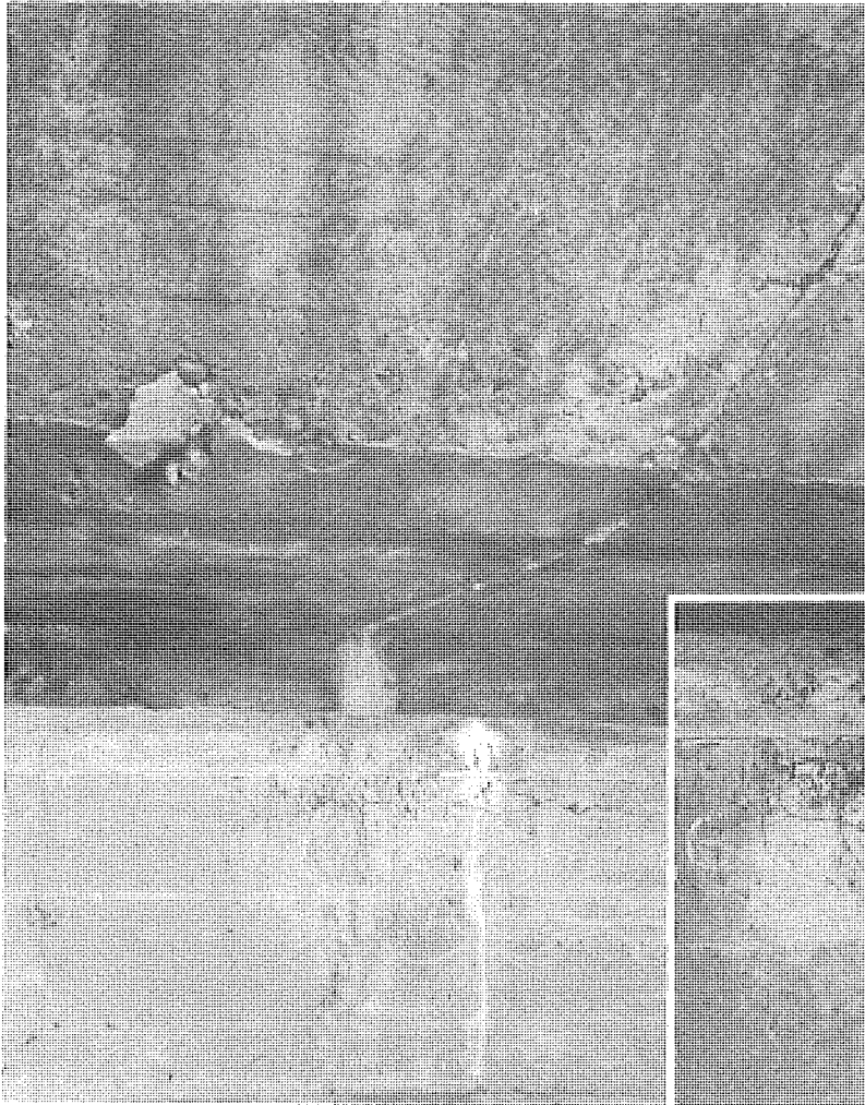
Figure 5. View of salt-afflicted area before and after investigation (mid-point of the center span on the west arch).
