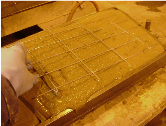
Wire mesh is placed in the filled form
