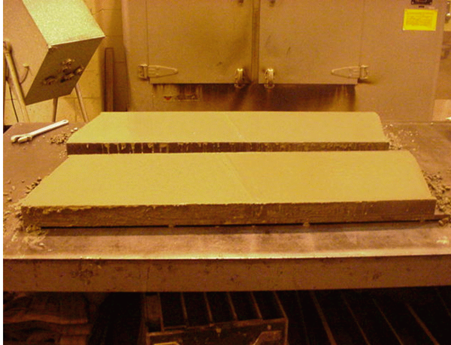
The remaining concrete is placed, consolidated, and struck off The slabs are then given a smooth finish with a steel trowel
