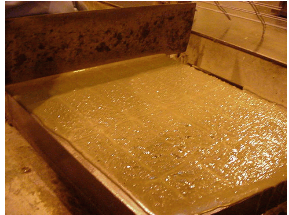
The excess concrete is struck off
