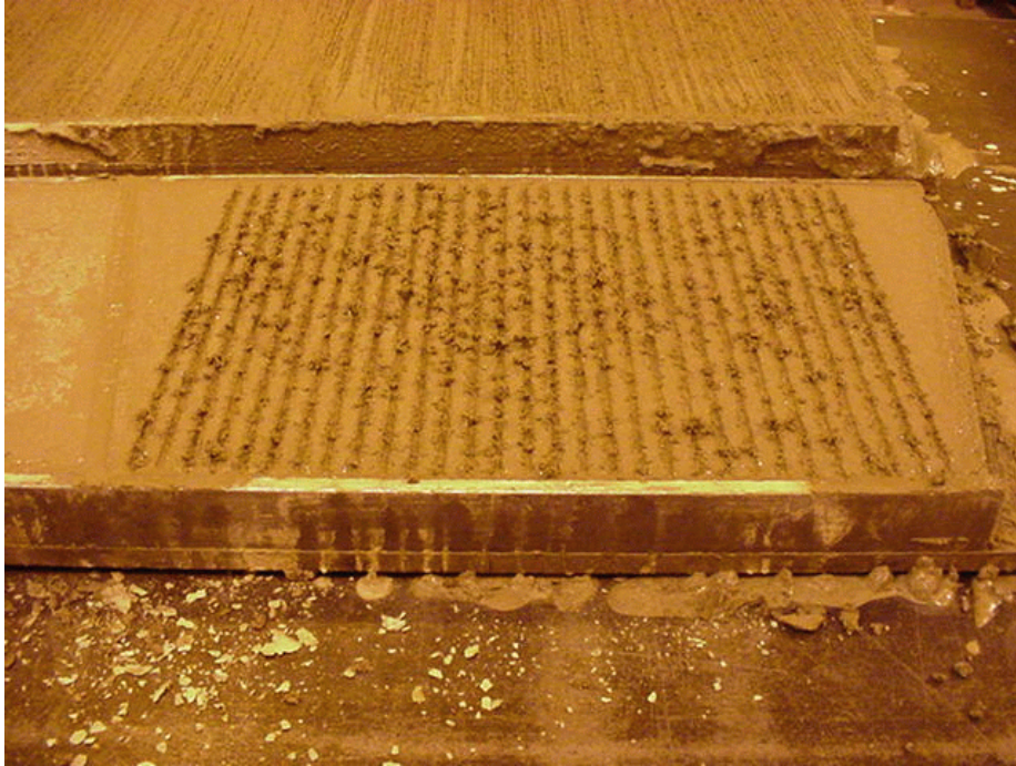
Transversely tined surface
