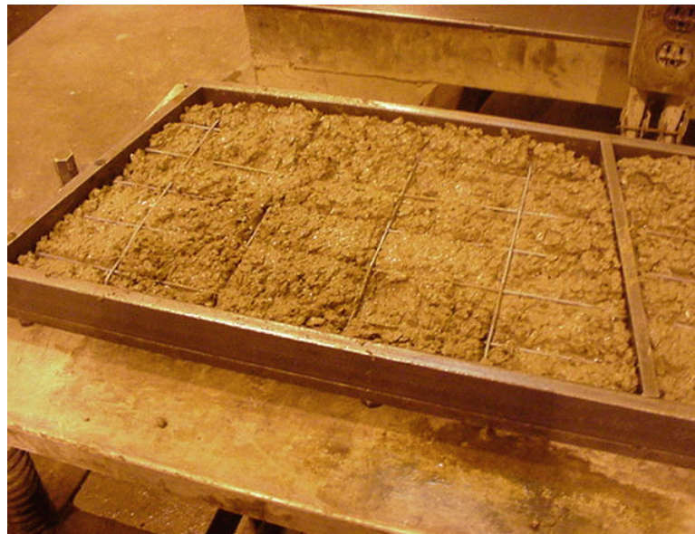
Wire mesh is placed on the first layer of concrete
