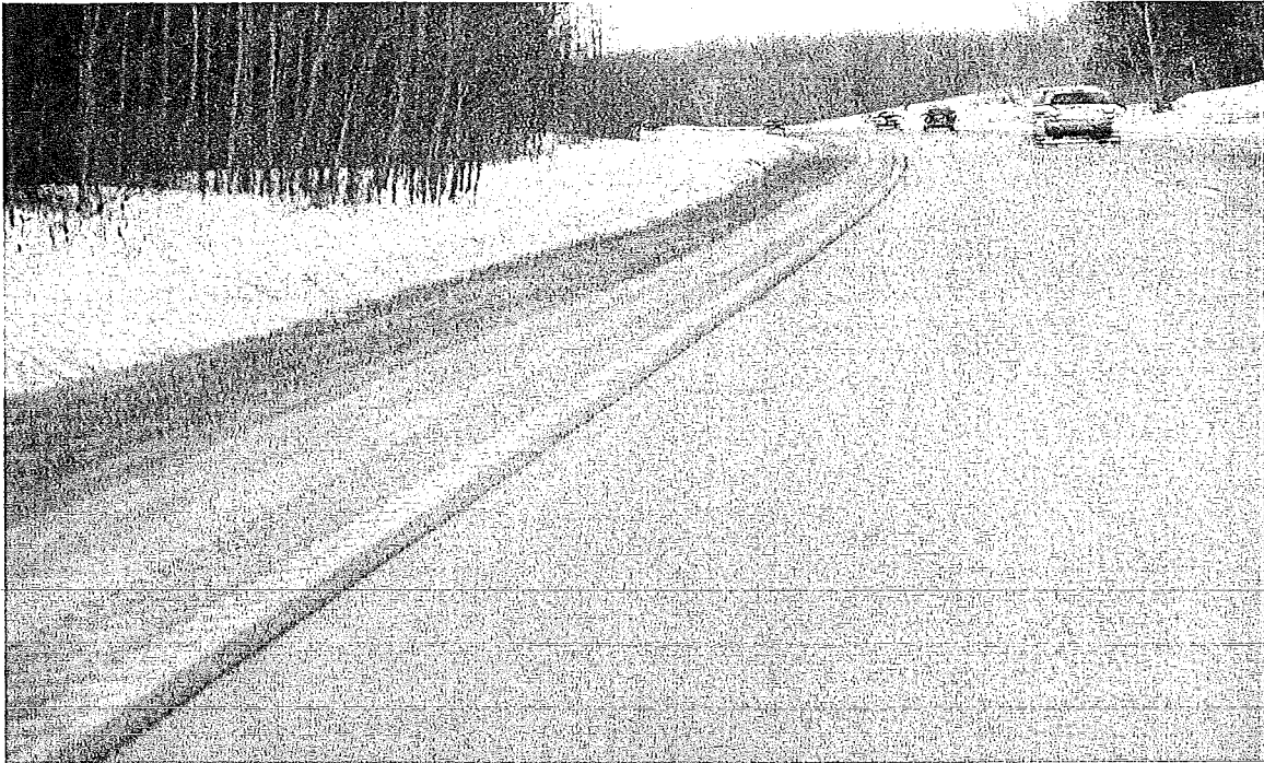
Figure 39. Performance of yellow 6-in rumbled edge line on Northbound US-131 after winter maintenance, February 15, 2004.
