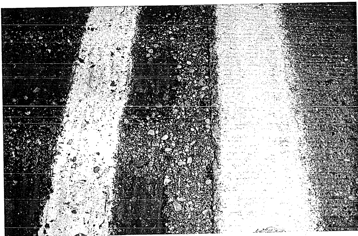
Figure 30. Close-up photo of 4-in white rumbled and white solid edge lines on Westbound I-96 after winter maintenance, April 25, 2004.
