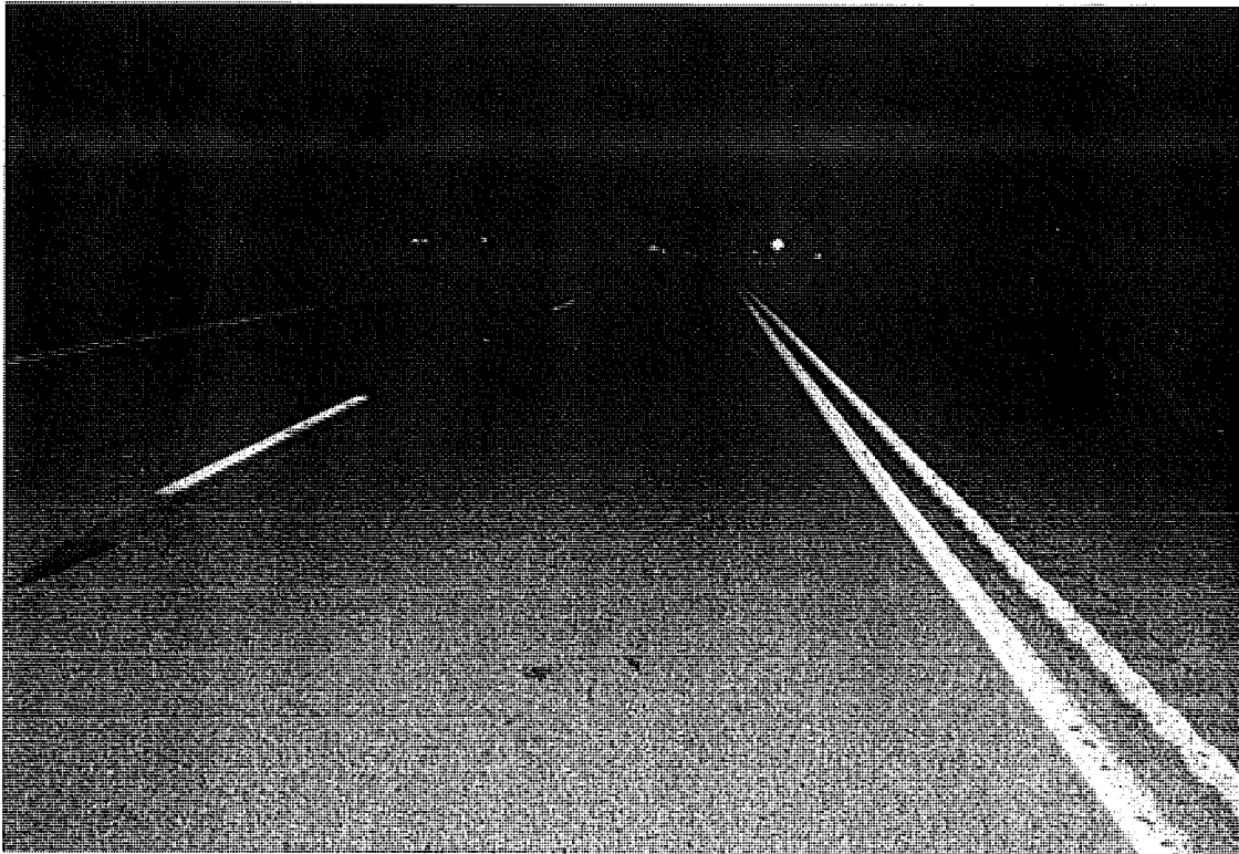
Figure 51. Night-time performance of white 4-in rumbled and solid edge lines on Southbound US-31 after winter maintenance, April 22, 2004.
