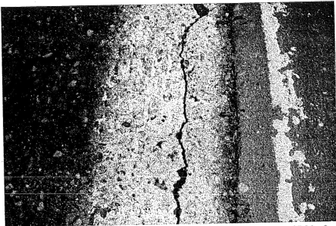
Figure 29. Close-up photo of 6-in white rumbled edge line on Eastbound I-96, after winter maintenance, April 25, 2004.
