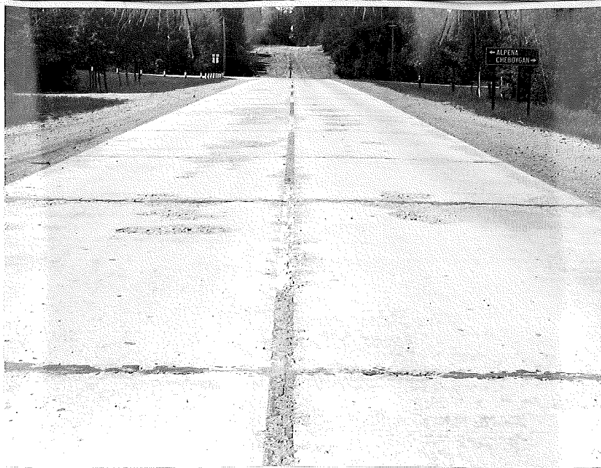
Fig. 6 F 71-24, C1 - Typical scaling at west end of project between Stations 30+20 and 37+00 where HP-7 was omitted.
