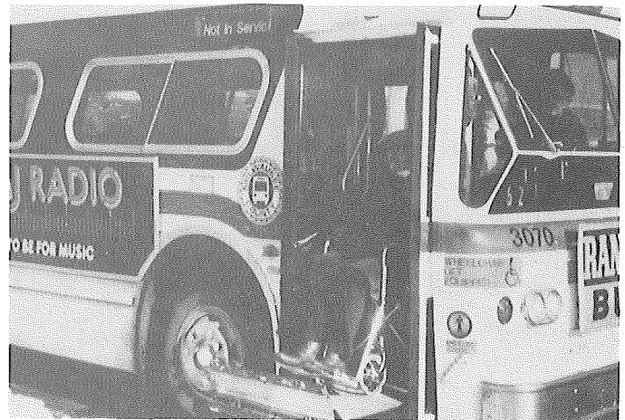
Step Lift in Front Door of Large Transit Vehicle
