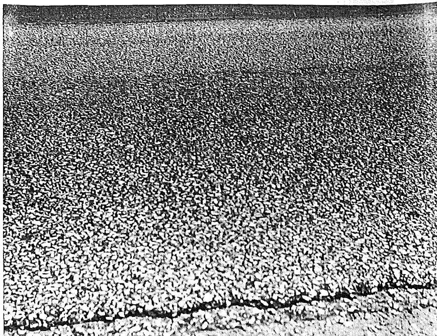
A. Typical condition of surface. No pitting.
