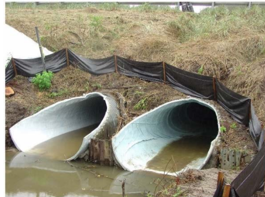
Cured in place (CIPP) liner
