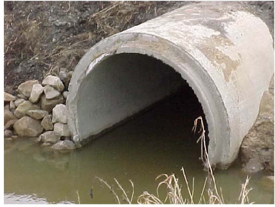
Example of concrete culvert
