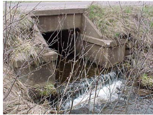
Headwall with wingwalls
