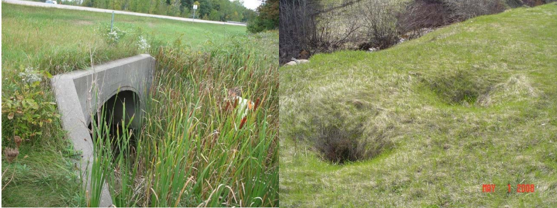
Embankment in same condition as design - condition rating of 8 or higher.
