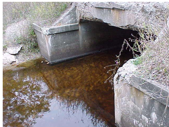
3-sided (no floor in culvert)
