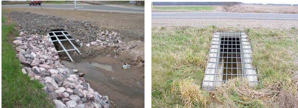
Examples of safety grates on culverts
