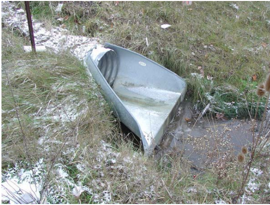
Example of metal culvert
