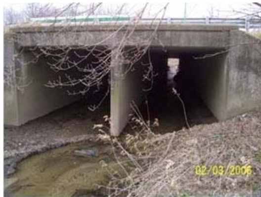
Example of a single culvert with 2 barrels (collect each barrel separately)
