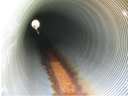
Condition rating 7 or
