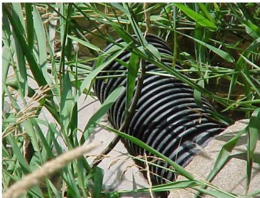
Concrete culvert with plastic liner
