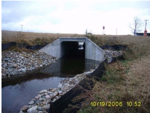
Riprap condition rating of 9. Riprap in same condition as initial placement
