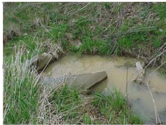
Concrete end section
