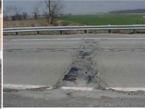
Condition rating: 6 or 7
