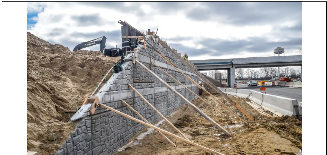
Permanent Mechanically Stabilized Earth(MSE) Walls
