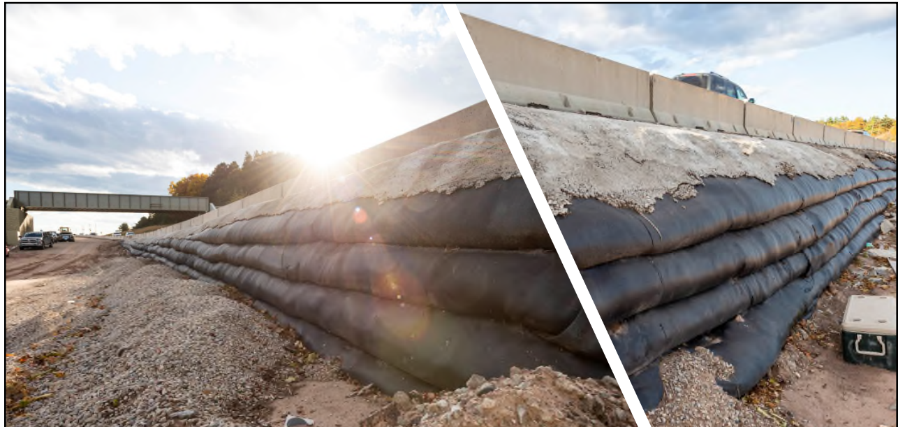
Temporary Mechanically Stabilized Earth(MSE) Walls
