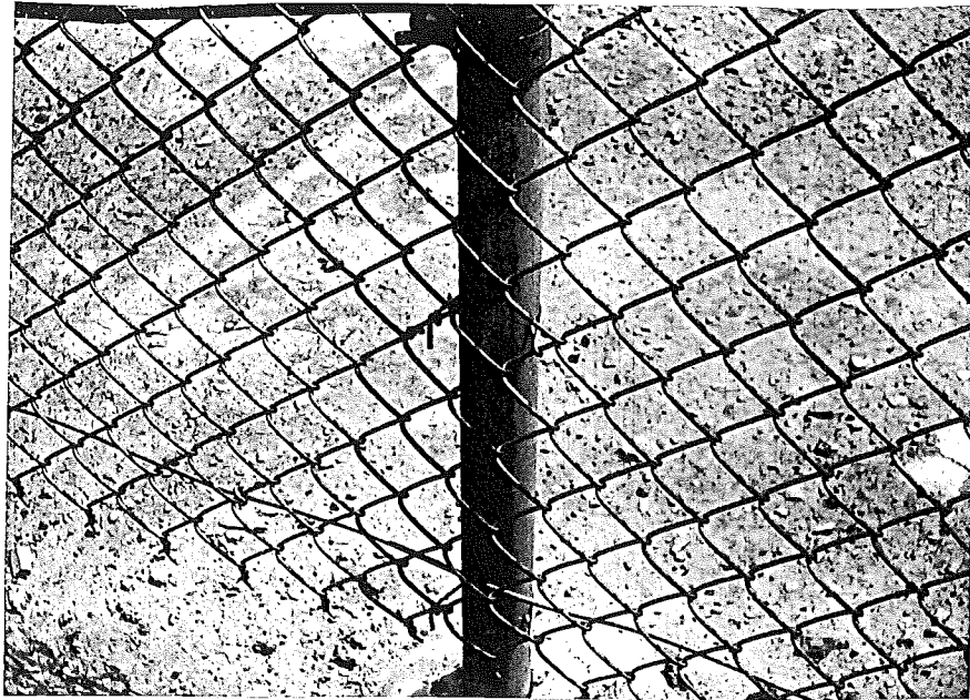
Figure 3. Aluminum fence; note incomplete wrapping of fabric tie at center of post.
