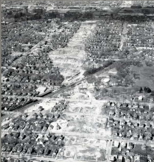
Clearing for I-196 in Grand Rapids
