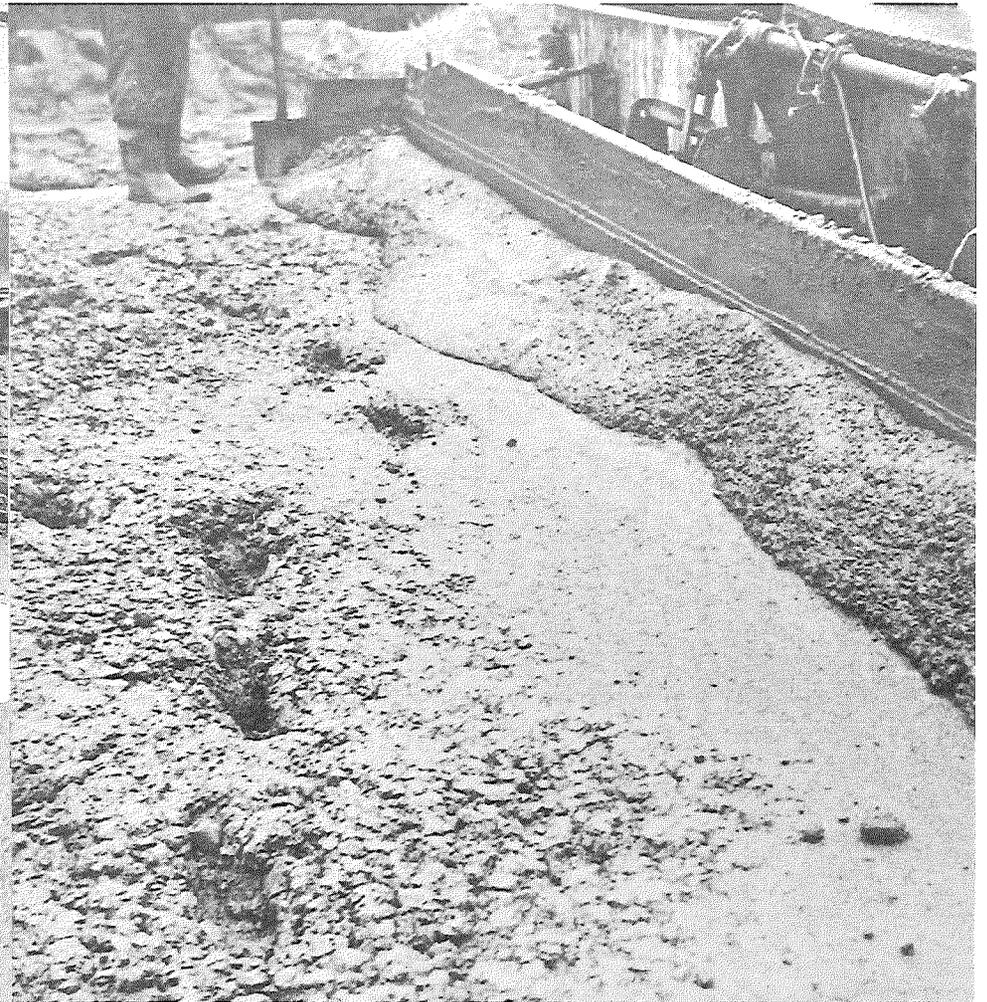
▲ Figure 24. Typical appearance of air-entrained concrete.
