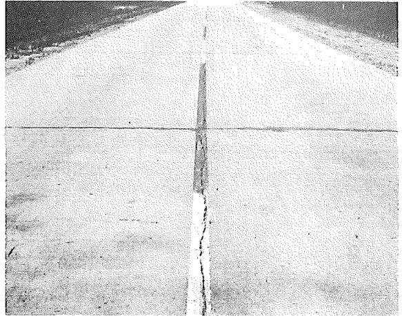
Broom finish, cutback asphalt curing
