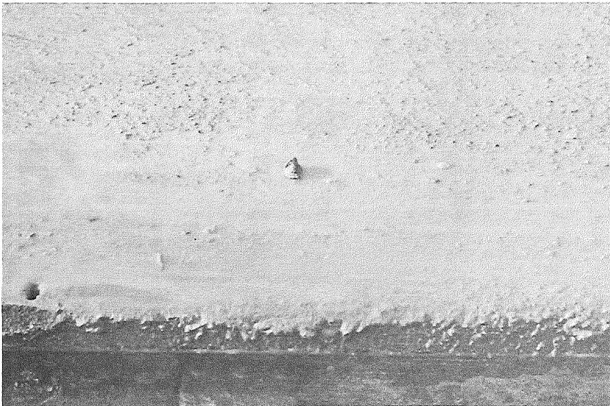
◀ Figure 25. Bleeding of concrete containing limestone fine and coarse aggregates.
