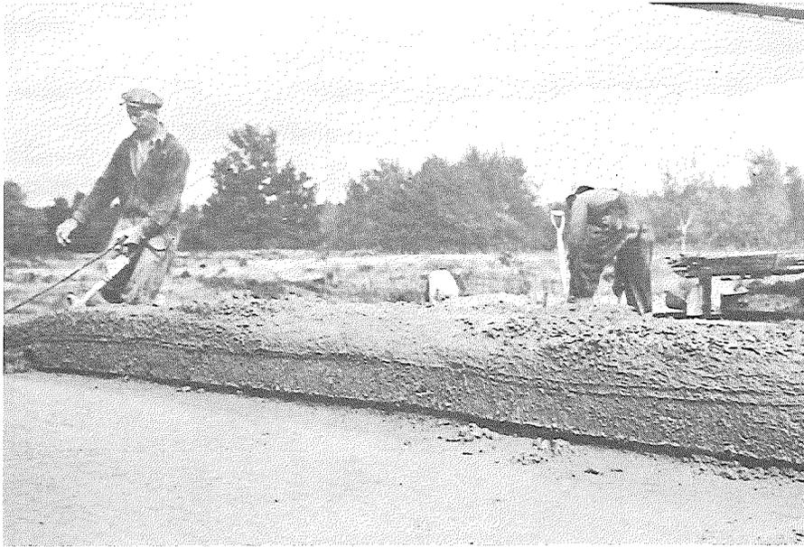
▲ Figure 23. Typical appearance of concrete containing added fines.
