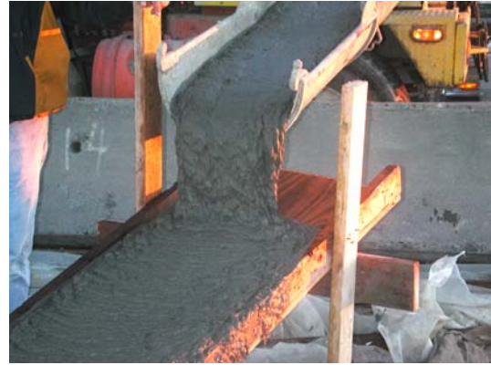
Figure 6.35. Flowability of ECC material discharging from truck.
