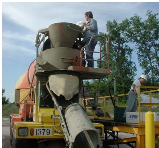
Figure 5.7. Adding fibers to truck.
