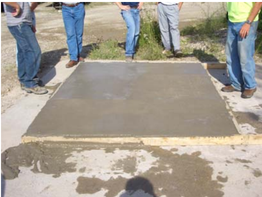
Figure 5.12. Finished ECC surface after steel troweling and tining.
