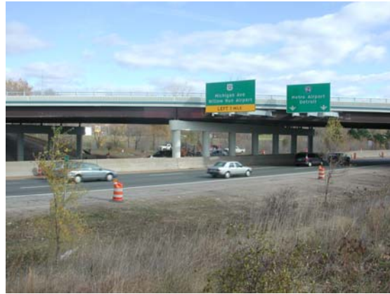
Figure 8.4 Completed Grove Street Bridge – elevation view
