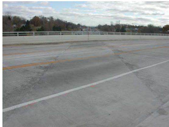
Figure 8.2 Completed ECC Link Slab
