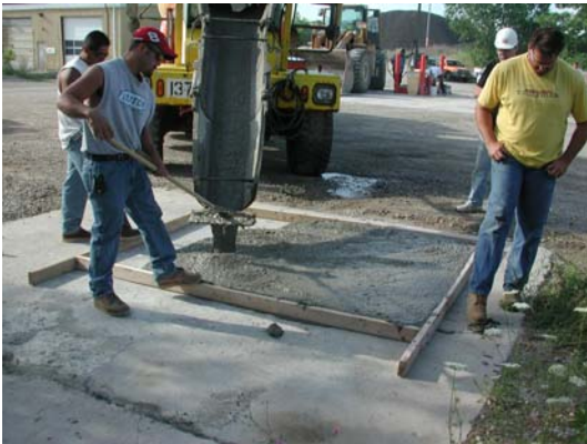
Figure 5.10. Placement of ECC into demonstration formwork.
