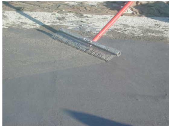
Figure 6.39. Tining of ECC link slab riding surface.
