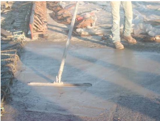
Figure 6.38. Steel trowel finishing of ECC link slab surface.
