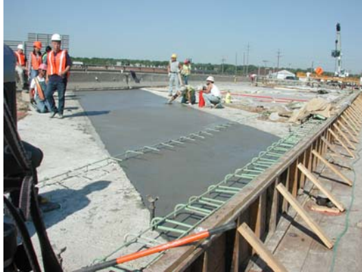
Figure 6.11. Hand finishing of ECC link slab riding surface.
