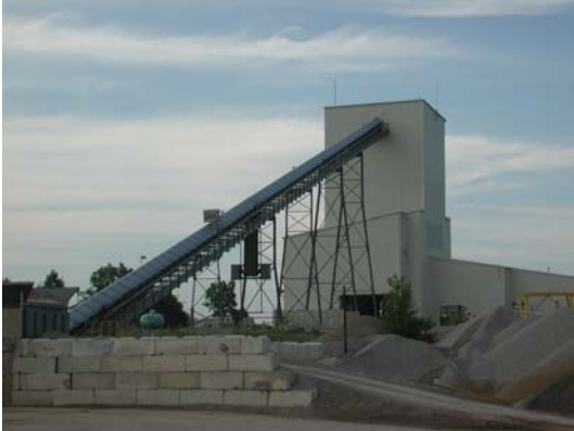
Figure 5.4. Clawson Concrete batching plant in Scio Township, Michigan.
