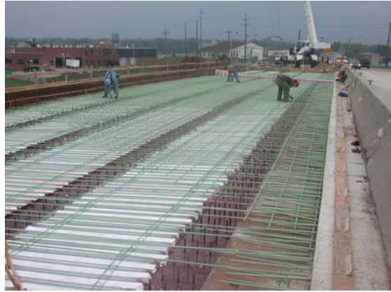
Figure 6.30. Installation of reinforcing steel.
