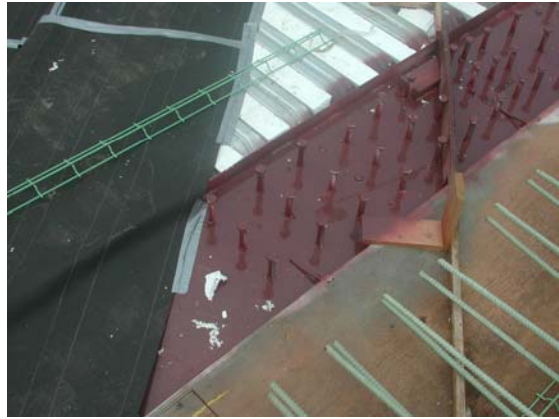
Figure 6.32. Shear connectors within debond zone and debonding layer (roofing paper).
