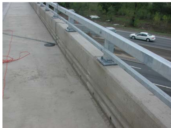
Figure 6.48. Completed concrete barrier wall and sidewalk.
