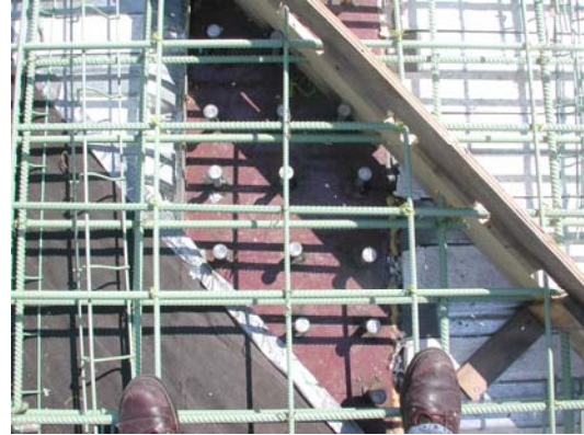
Figure 6.6. Shear developers in link slab transition zone.
