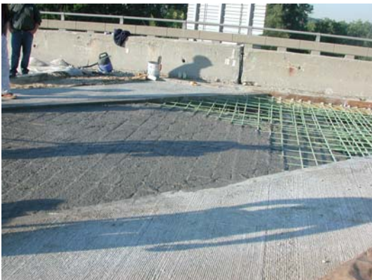
Figure 6.9. ECC material flowing throughout link slab confines.
