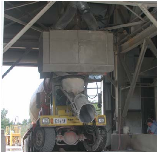
Figure 5.6. Charging concrete truck with sand, fly ash, cement, water, and high range water reducer.
