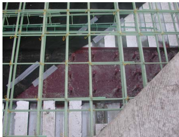
Figure 6.33. ECC link slab transition zone with completed adjacent concrete deck.
