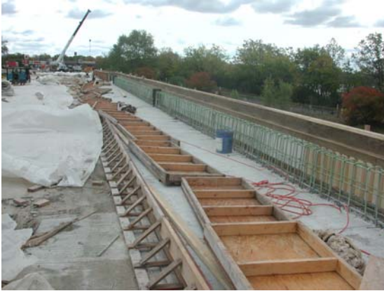
Figure 6.45. Construction of concrete sidewalk and barrier wall.
