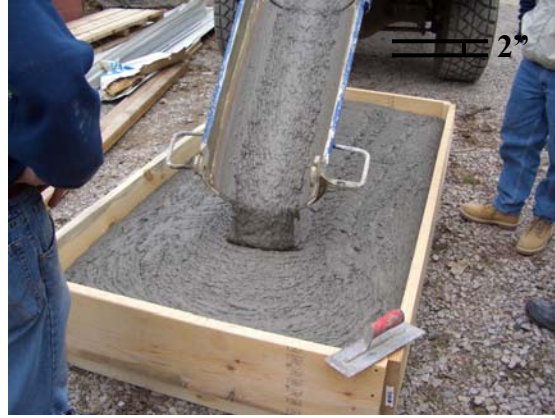
Figure 4.26 ECC Filling Formwork
