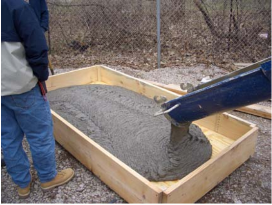
Figure 4.25 ECC Pouring into Formwork
