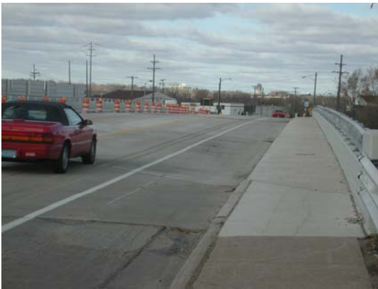
Figure 8.1 Completed Grove Street Bridge – deck view
