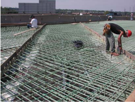
Figure 6.5. Completing installation of continuous reinforcing steel throughout ECC link slab.
