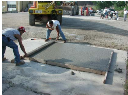
Figure 5.11. Screeding of ECC surface.
