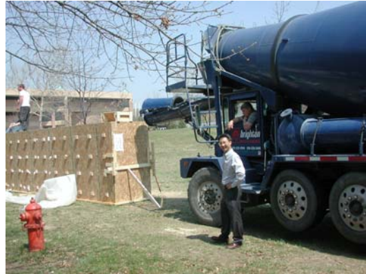
Figure 4.15. Delivery of ECC to jobsite
