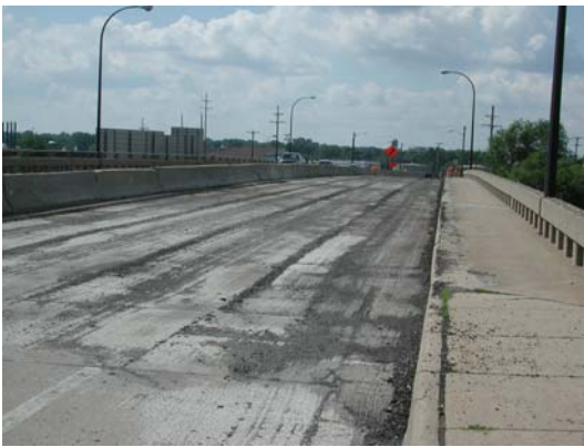
Figure 6.1. Removal of bituminous asphalt wearing surface.
