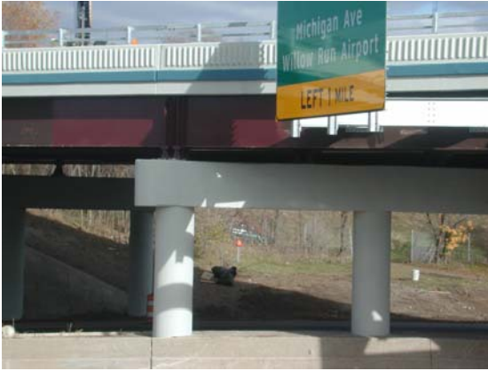
Figure 8.3 Grove Street Pier Two Under Completed ECC Link Slab
