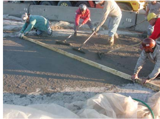
Figure 6.37. Screeding of ECC link slab finished surface.
