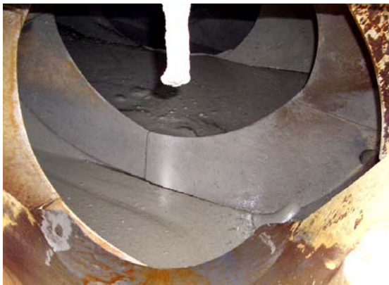
Figure 4.12. Creamy ECC Mortar Matrix
