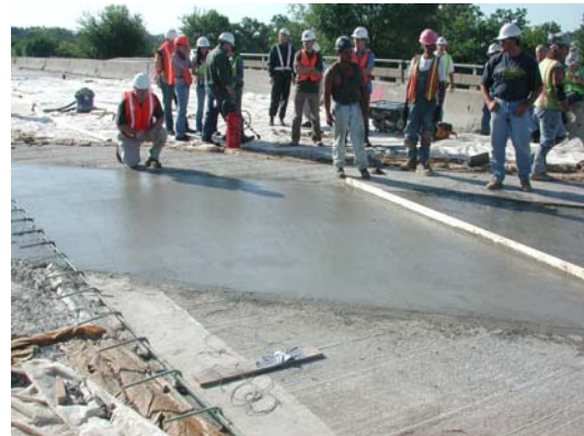
Figure 6.10. Screeding of ECC material to final surface grade.
