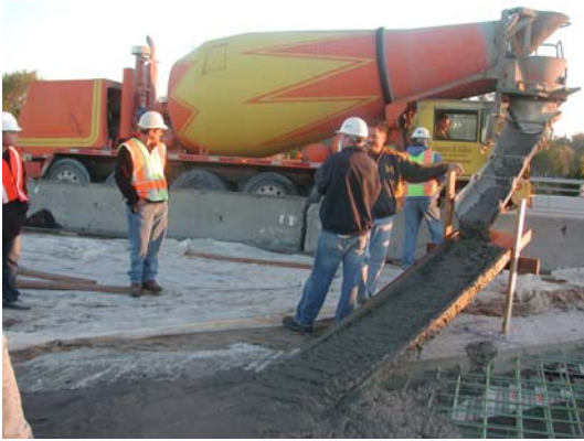
Figure 6.34. Placing of ECC material at the link slab location – phase two
