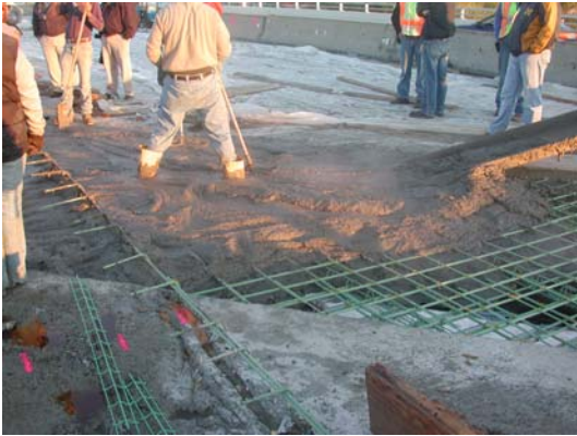
Figure 6.36. Placing of ECC material at the site – phase two
