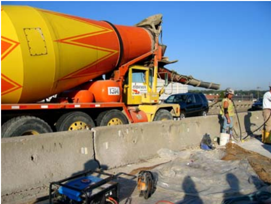
Figure 6.7. Arrival of ECC material in concrete mixing truck.
