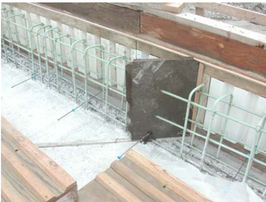
Figure 6.47. Expansion joint within concrete barrier wall and sidewalk.
