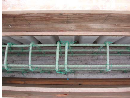
Figure 6.46. Reinforcement detailing within concrete barrier wall.
