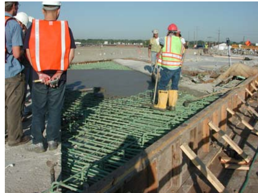
Figure 6.8. Placement of first truck of ECC material at link slab location.
