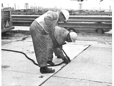
Joints are sealed with hotpoured rubber-asphalt sealant.
