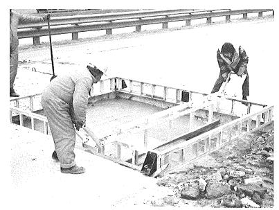
A mortar base is poured and struck-off to the proper elevation.
