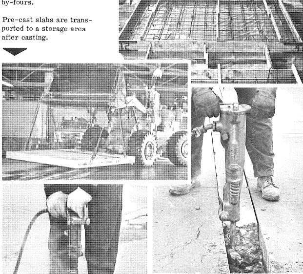
After the full-depth sawing of the pavement, the concrete is removed between the narrowly spaced saw-cuts.
