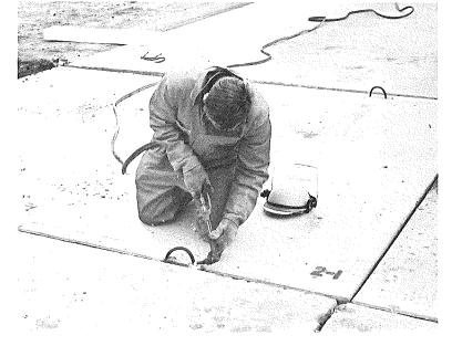
Premolded bituminous impregnated filler board is installed (slotted board used with doweled joints).
