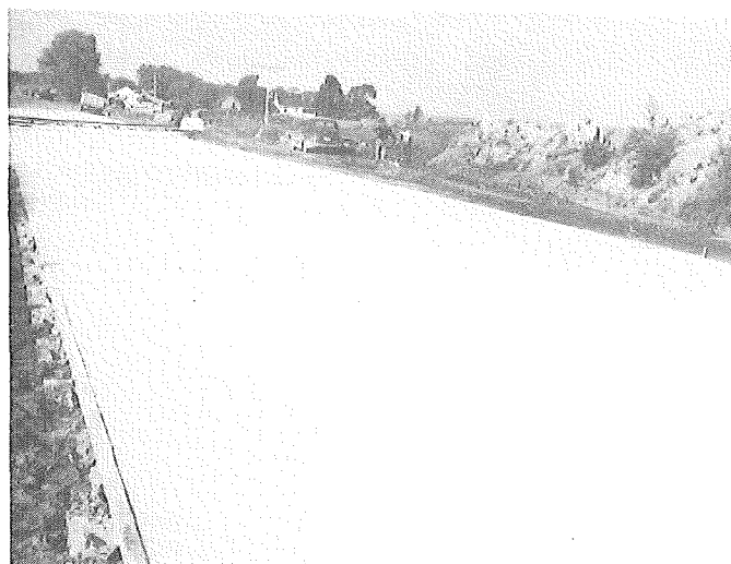
▲ FIGURE 3. APPLICATION BY DOUBLE PASS WITH NOZZLE SCREENS REMOVED AND SPRAY BAR SLIGHTLY RAISED.
