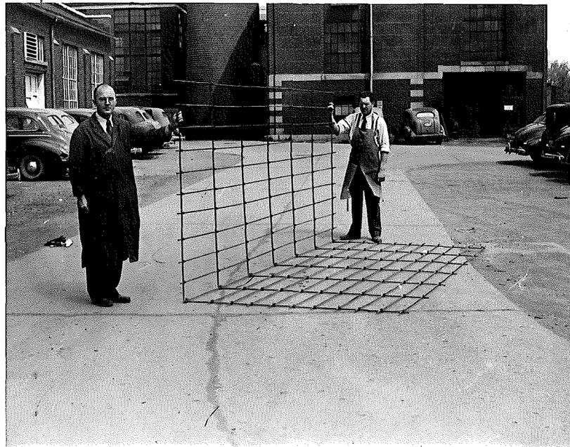
Figure 3. Unfolding hinged mat.
