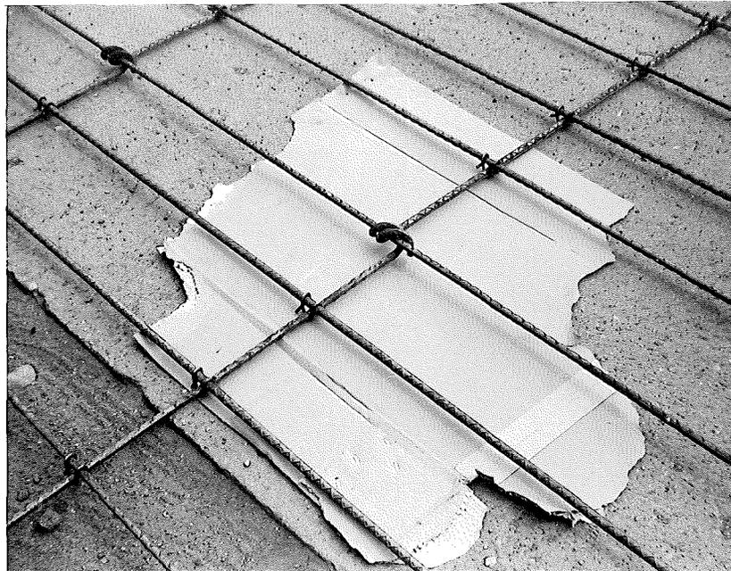
Figure 4. View showing how hinge is fabricated.
