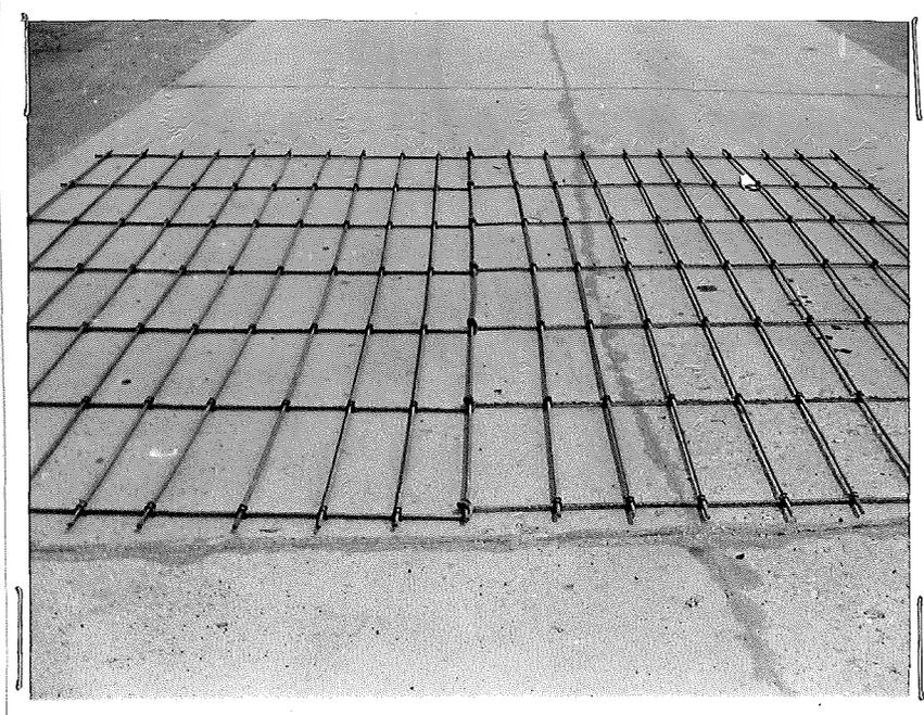
Figure 1. View showing hinge construction in center of mat.
