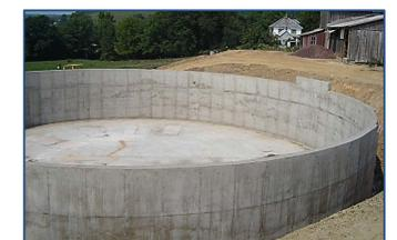
Precast Concrete Retaining Wall
