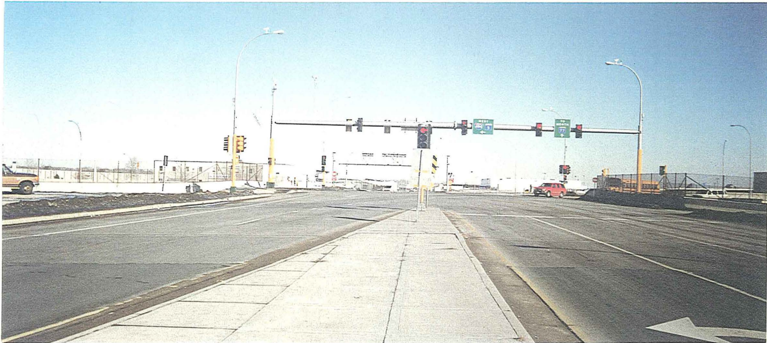
Figure 5: SPUI with cross-road going over the freeway with all signal heads located on a single overhead tubular beam.
