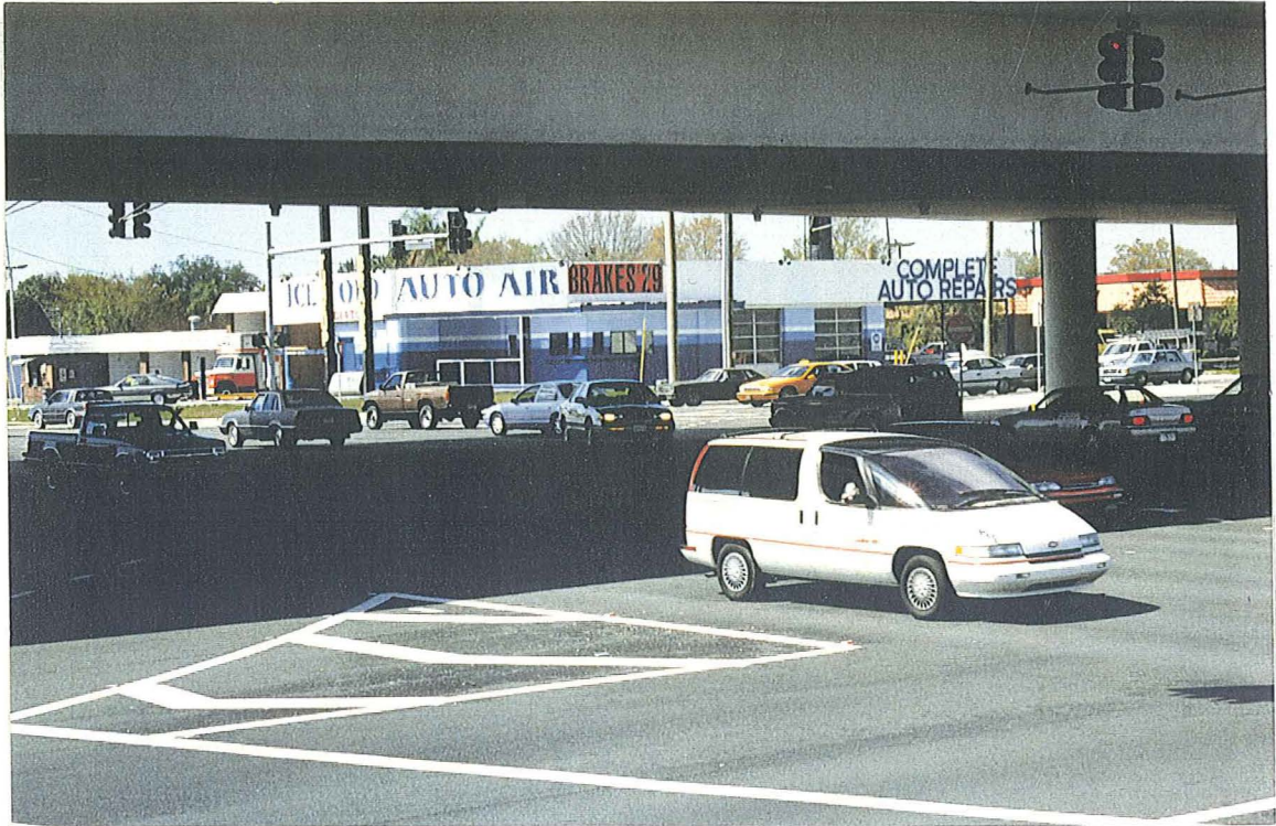
Figure 6: Confused driver (car with lights on) stopped in middle of a SPUI while traffic proceeds on either side
