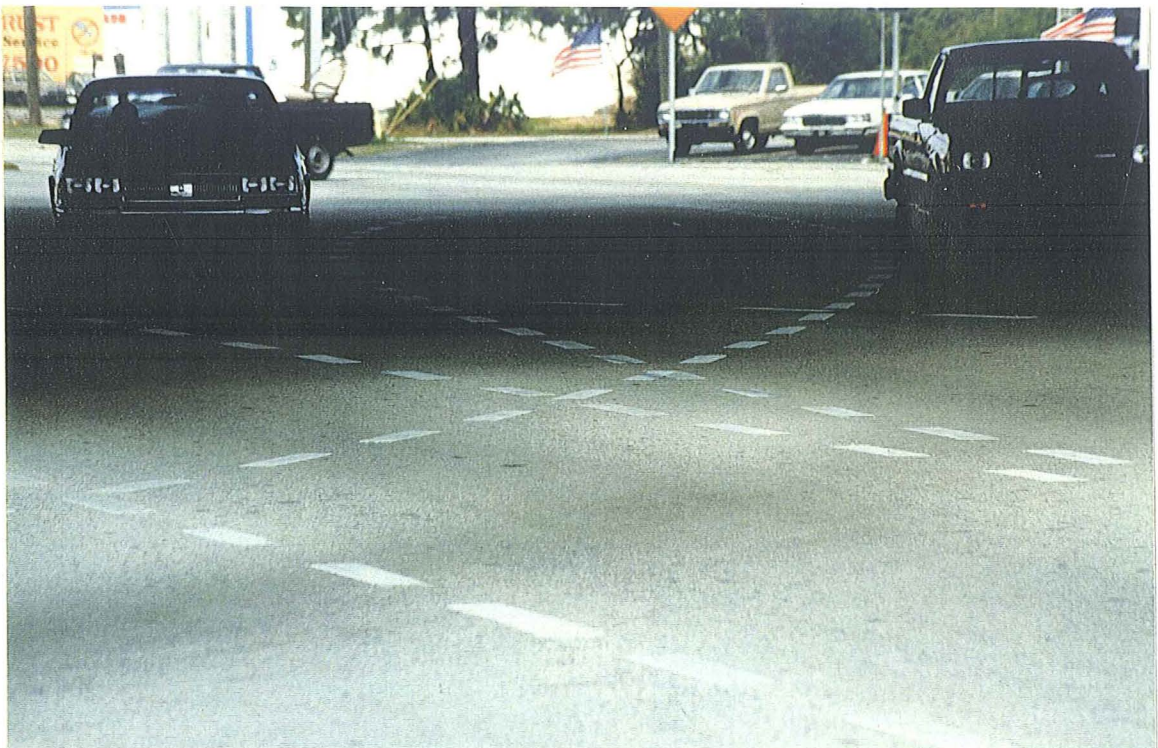
Figure 9: Pavement marking overlap creates driver confusion
