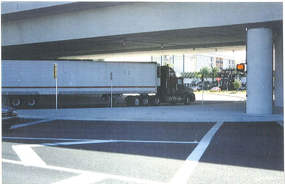
Figure 7: U-turn lane accommodates large trucks
