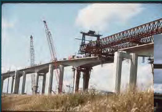
➤ Rotation of cantilevers 11N & 11S
