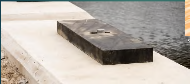
Elastomeric bearing on an abutment
