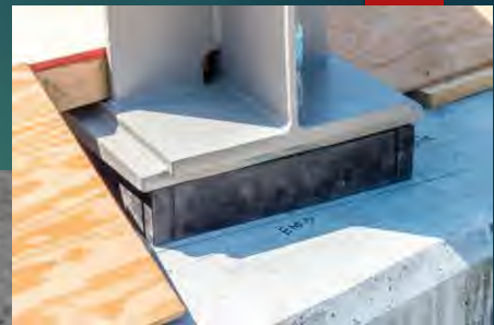
Steel beam on an elastomeric bearing
